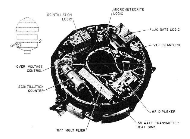
Figure 9. Able-3 Payload (Bottom View).
