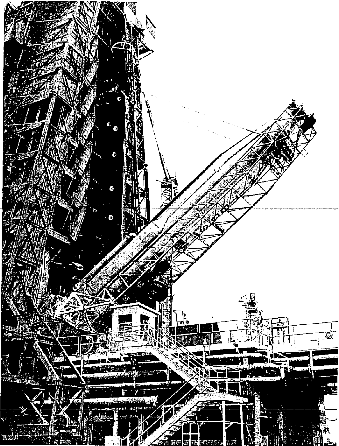
Figure 1. Installation of Atlas 80D on Pad 12. Note how Launcher Mechanism Tilts to Mate with Atlas Handling Trailer.
